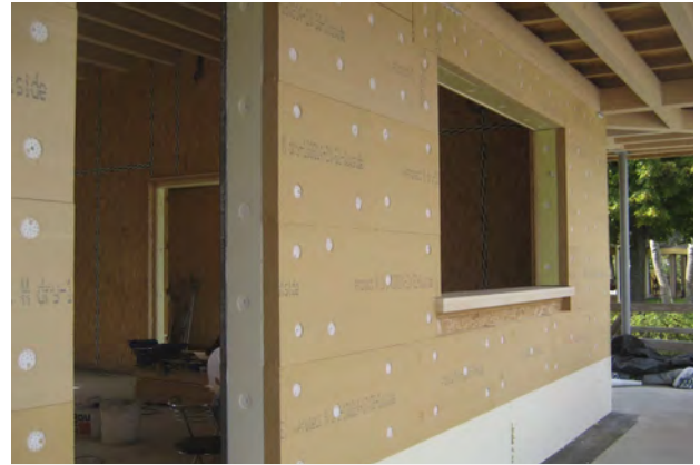
The thermal insulation system is recommended both in new buildings and in renovations. It improves the energy performances and allows the rooms usability during installation.
